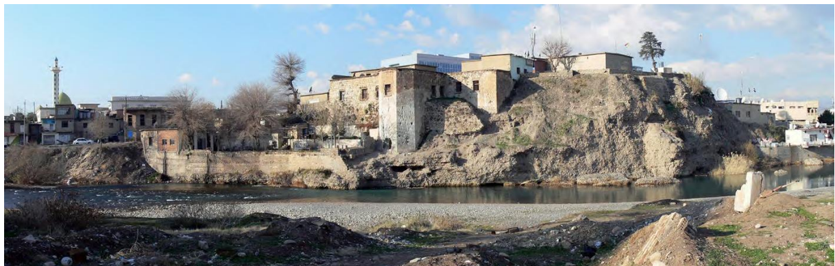
Fig. (6): Zakho Castle today (source: Zakho master plan report (Duhok Municipalities Directory, 2011))
