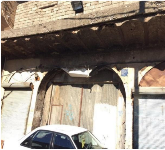
Fig.(4): House in Old bazar street Figure
