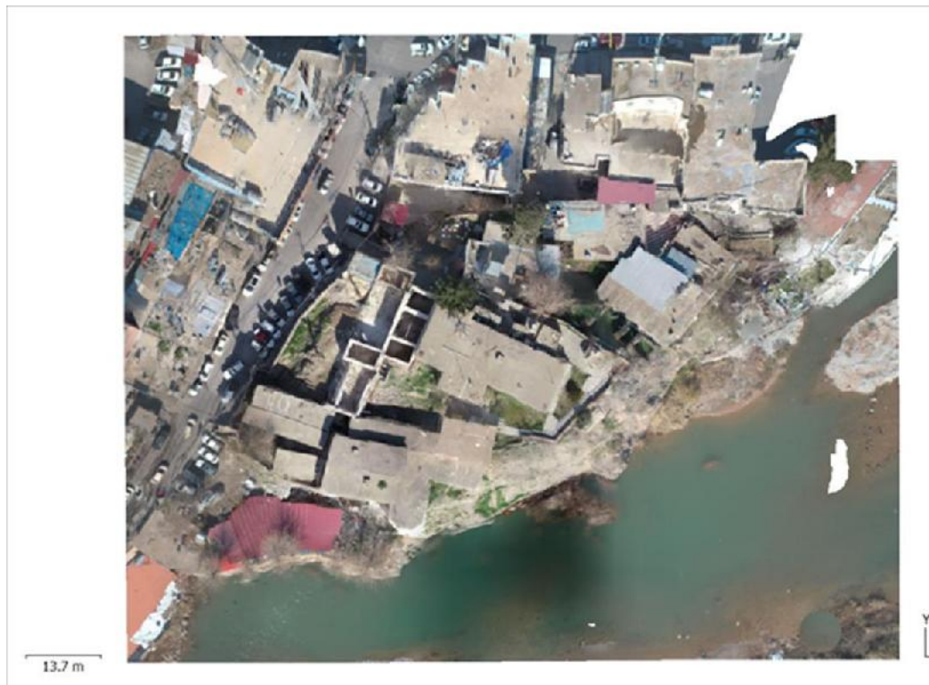
Fig.( 10):- Orthomosaic of Qishla Building
