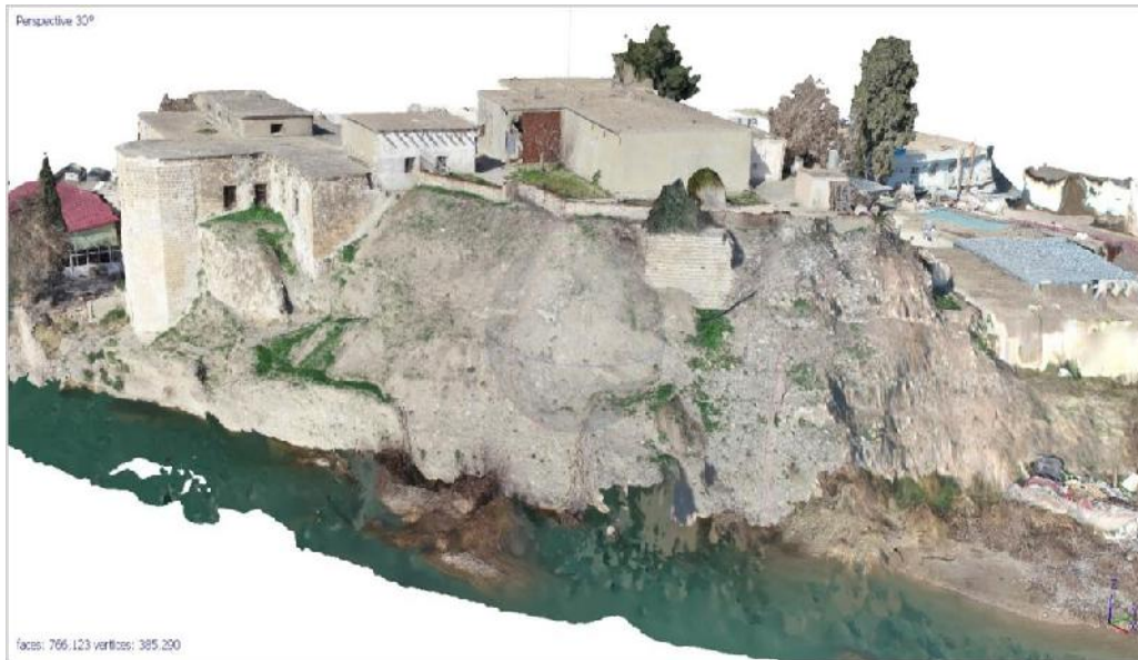
Fig.(12 ):-B: 3D Model of Qishla Building from East Side (Khabour River)
