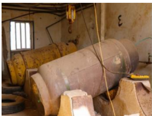
Fig.( 4): -Chlorine gas cylinders
