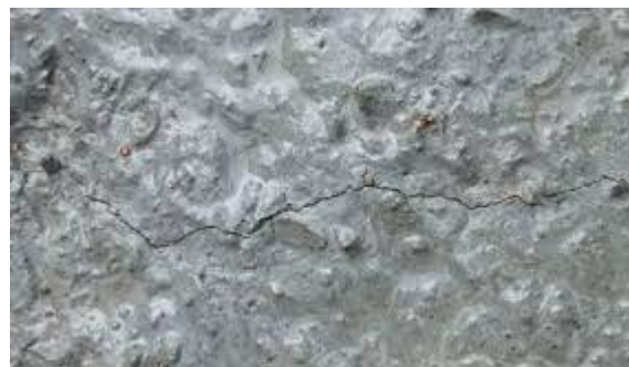
Fig.( 10):- Autogenous Shrinkage Cracks [28].
