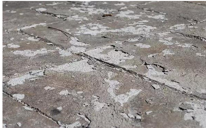
Fig.( 9):- Freezing and thawing cracks [27].
