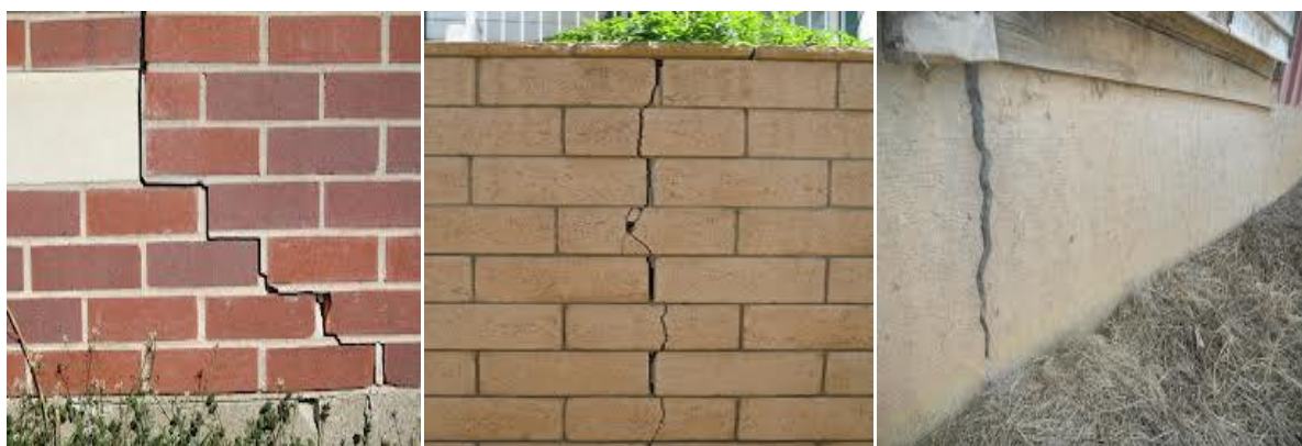
Fig.( 5):- Cracking due to movement or settling of the ground [24].
