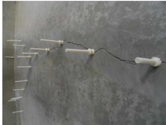
Fig.( 1):- Epoxy injection [45].
