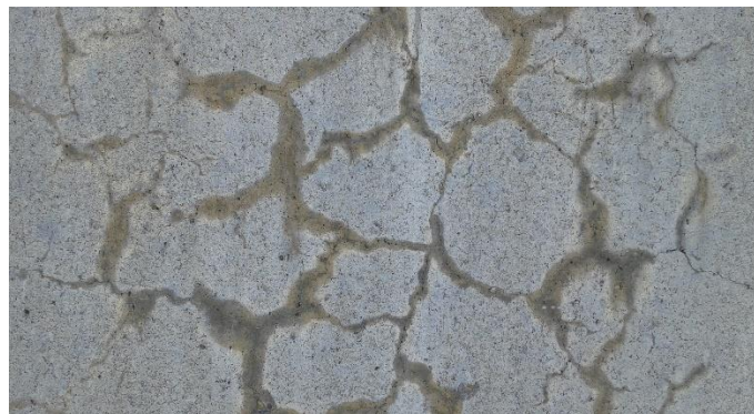
Fig.( 8):- Alkali-aggregate reaction [1]
