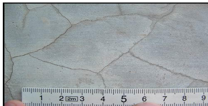
Fig.( 11):- Crazing crack [29].
