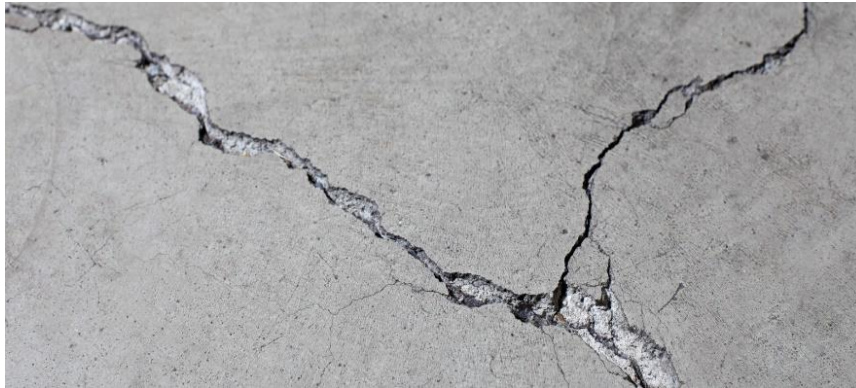
Fig.( 7):- Sulphate attack cracks [1]
