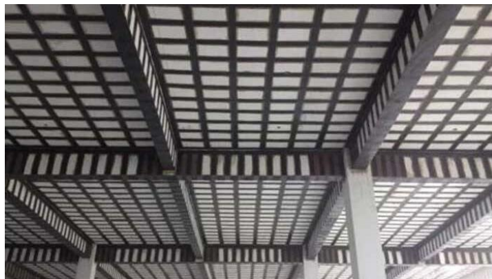
Fig.( 4):- Repairing cracks using CFRP composite [51].
