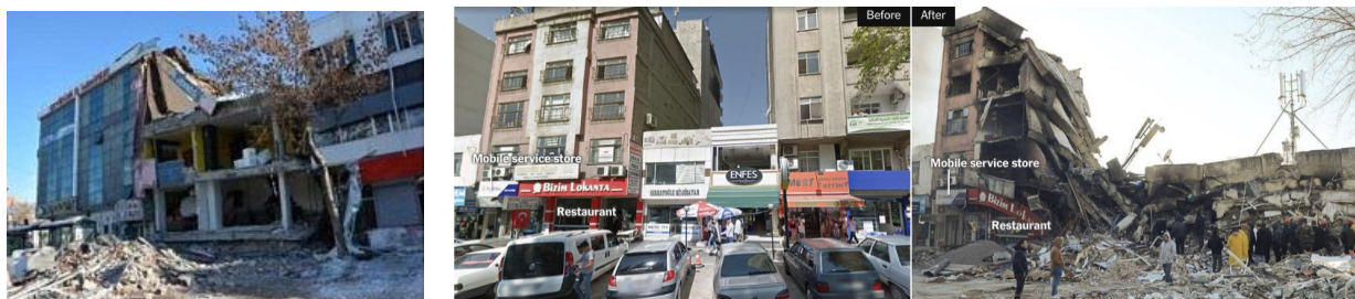
Fig.( 15):- Damage and collapses of buildings due to pounding effects (Alhawamdeh et al., 2023; OZTURK et al., 2023).
