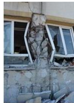
Fig.( 7):- Damage due to the short column formation in some buildings (OZTURK et al., 2023).
