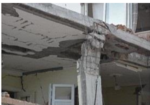
Fig.( 13):- Severe damage to RC buildings with infilled ribbed or flat slab (OZTURK et al., 2023).
