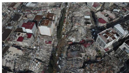
Fig.( 2):- Wreckages of destroyed buildings resemble heaps of sand and gravel (Lekkas et al., 2023; OZTURK et al., 2023).
