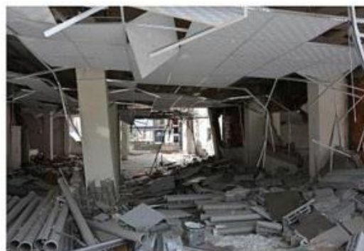
Fig.( 13):- Severe damage to RC buildings with infilled ribbed or flat slab (OZTURK et al., 2023).
