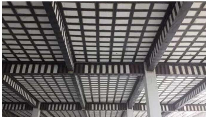
Fig.( 4):- Repairing cracks using CFRP composite [51].
