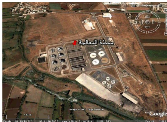
Fig.( 2):- Aerial view of the sewage treatment plant in Homs city
