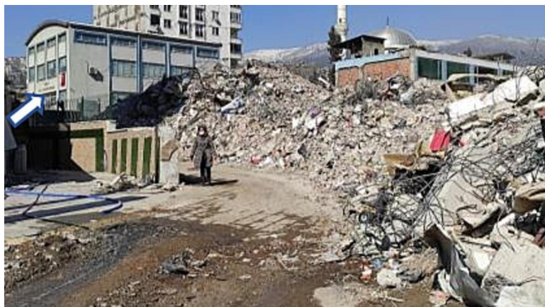
Fig.( 1):- The difference in the seismic response and damage of adjacent buildings, Kahramanmaraş (OZTURK et al., 2023).
