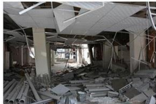
Fig.( 13):- Severe damage to RC buildings with infilled ribbed or flat slab (OZTURK et al., 2023).
