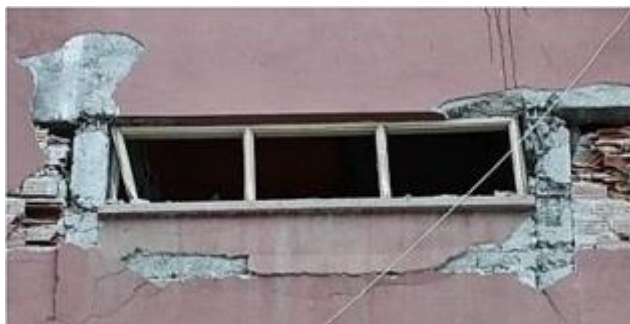
Fig.( 7):- Damage due to the short column formation in some buildings (OZTURK et al., 2023).
