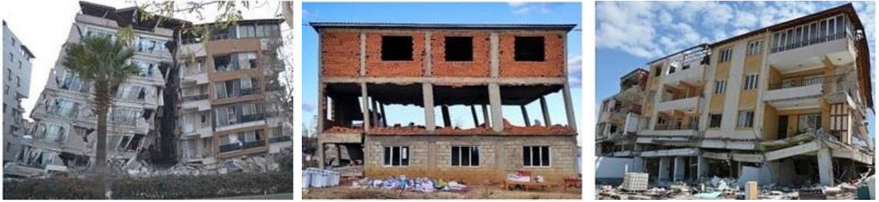
Fig.( 9):- Collapses resulting from soft or weak stories in RC buildings (OZTURK et al., 2023).
