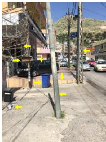
g) Power poles; garbage bins; parked cars; uneven level
