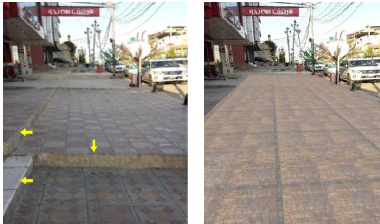
Fig. (5): Left –A sidewalk with sudden, vertical changes in level a commercial area; Right - Post-processing rendering of the same image ( Credit: The authors )
