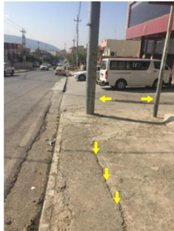
e) utility poles
