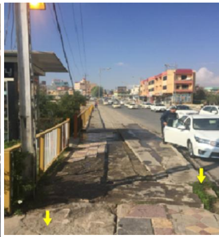
Fig. (9): Left - Sidewalk surface with pits & wide cracks Right - Rendering of the sidewalk after pavement (Credit: the Authors)
