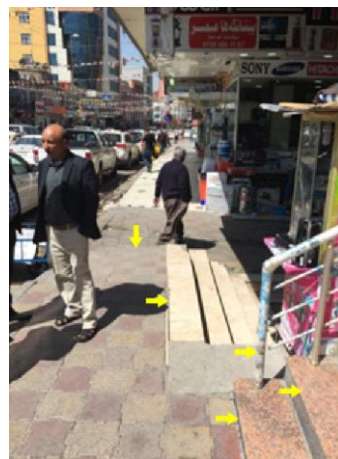
h) Sudden/unexpected descending steps
