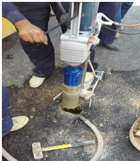
Fig. (5): Core taken from test road
