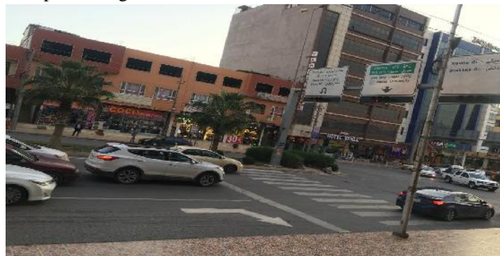
Fig.(9): Newly added white solid dividing line and right turn arrow, Bira intersection
