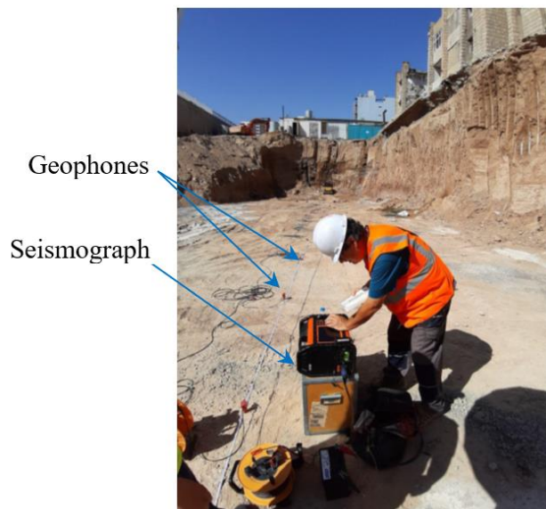
Fig. (4): The seismograph (Terraloc Pro) at the tower-building site, Erbil.
