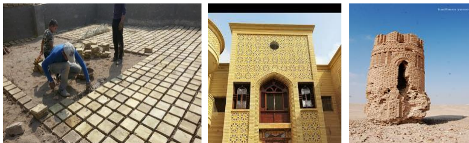
Fig. (3): Traditional clay bricks (Farshi) used for exposed tiling and other building purposes
