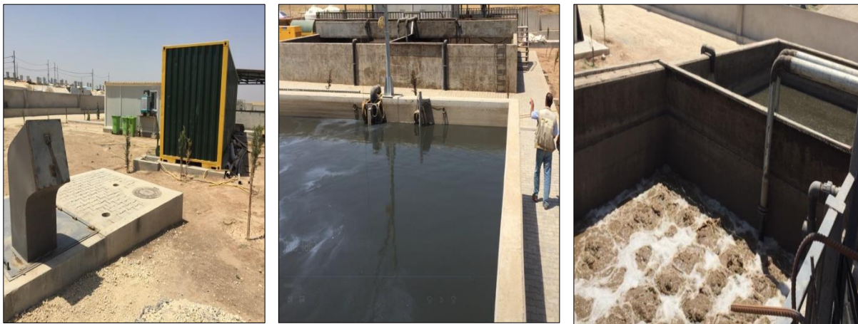
Fig. (6): Wastewater treatment plant of Kaparto2 IDPs camp
