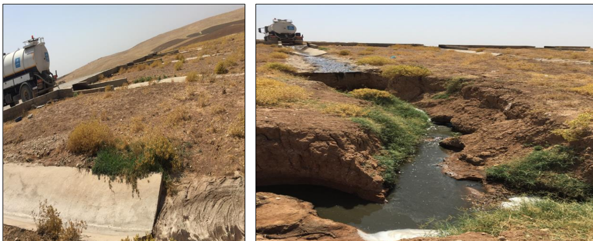
Fig. (8): Dumping the wastewater of Domiz1 refugees camp at open area
