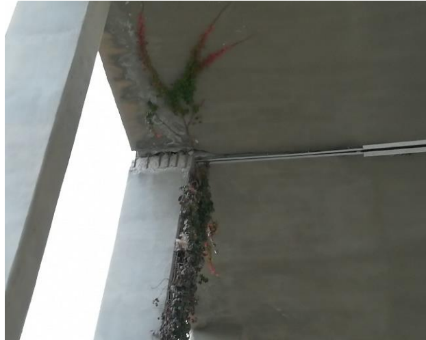
Fig. (8): Pounding effect between two columns in the Children Hospital in Halabjah
