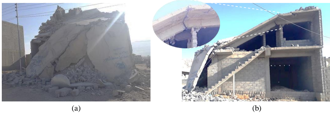
Fig. (15): (a) Front view of a collapsed three-story hybrid building (b) Side view of the same building
