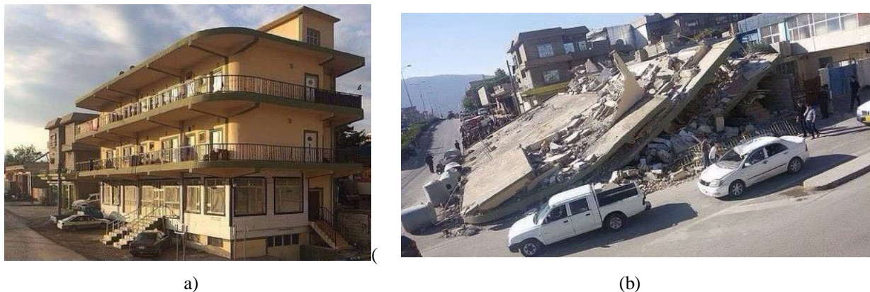
Fig. (19 (a)). The building before collapse. (b) Collapse of Four-story R.C frame Building.
