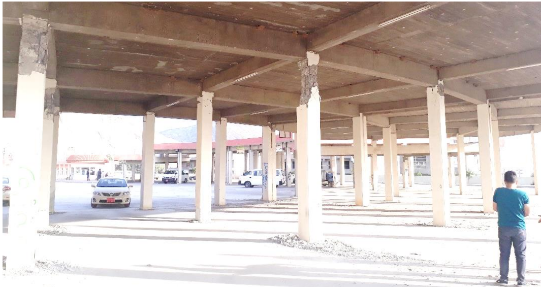
Fig. (22): Hinging in columns with an idea on the shape of the station
