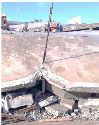
Fig. (10): Large R.C lintels of depth of more than one meter in front of the house
