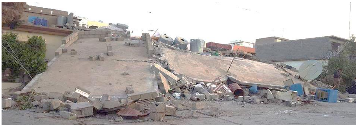
Figure 9. Collapse of a three-story Building using Hybrid system of (R.C Frame- Masonry) (front view)
