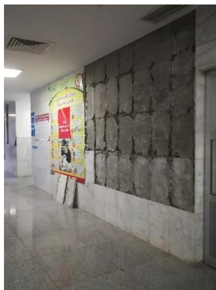
Fig. (7): Falling of heavy tile finishing inside the Children Hospital in Halabjah
